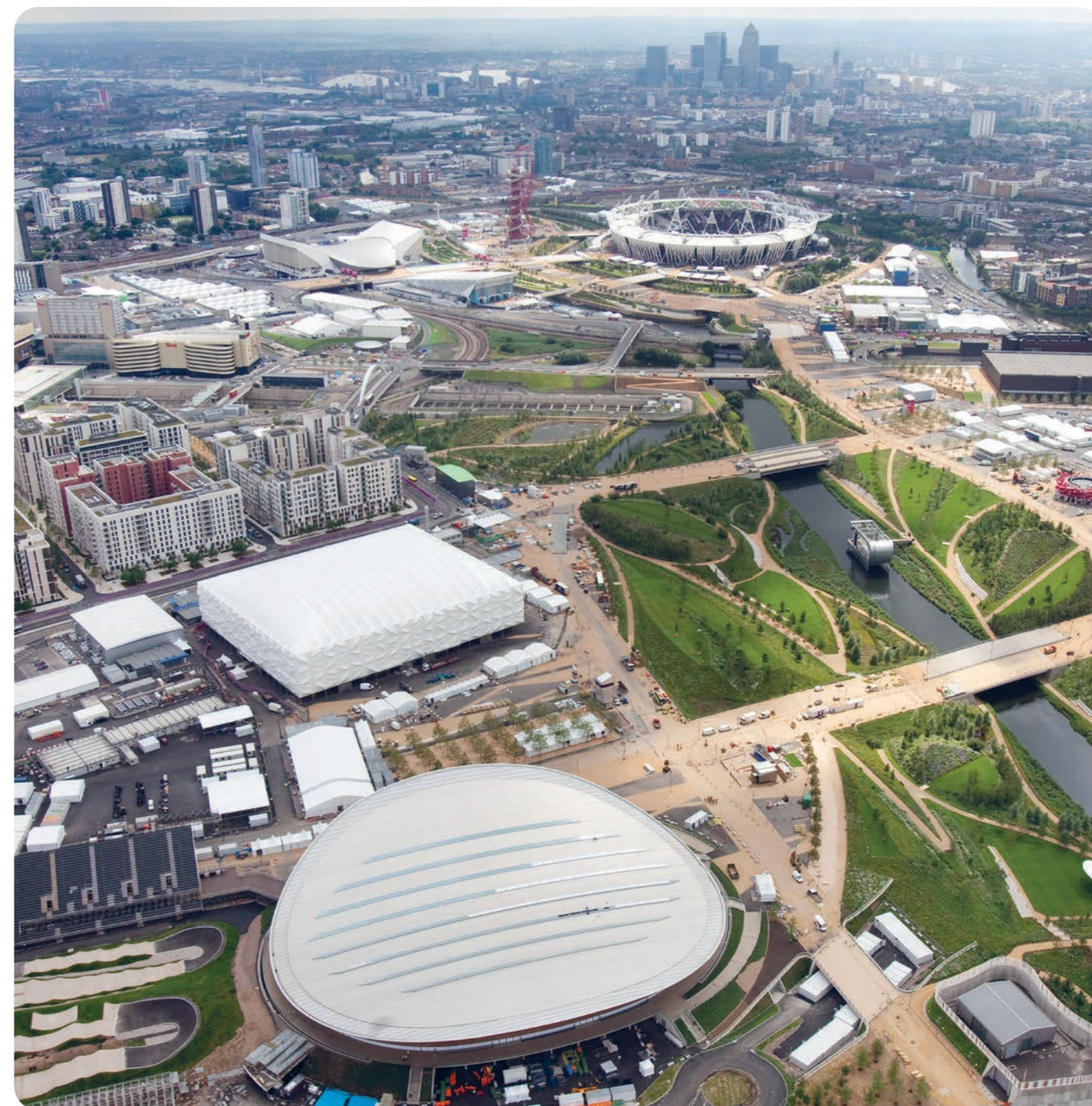
London 2012: aerial shot over Olympic Park.
